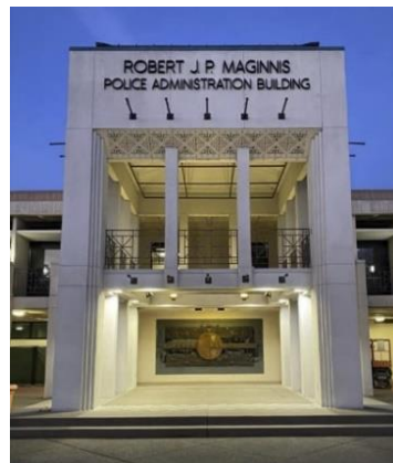
Fig. 2, Robert J.P. Maginnis, Police Administration Building, E14th Street, San Leandro
